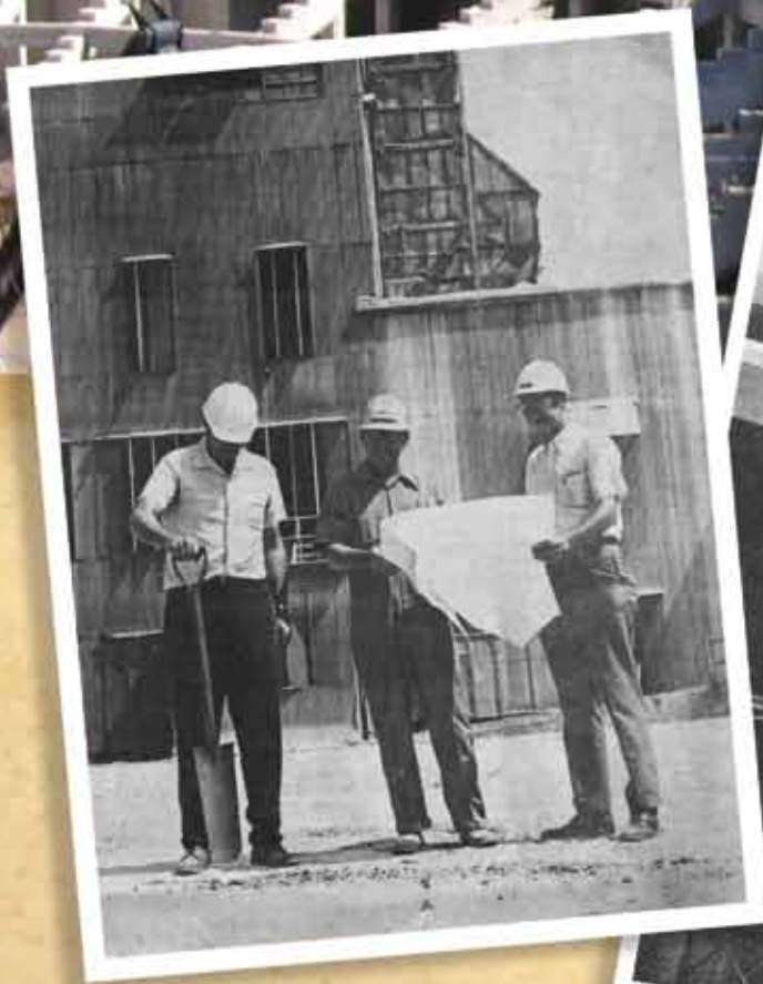
On July 24, 1972, Midwest Carbide Chief Engineer Bob Scherrer breaks ground while Chuck Williams of Williams Construction and Ed Sexton, Midwest Carbide Plant Superintendent review plans for a new dust collector system. The shovel was the same one used for the original plant groundbreaking in 1953.
