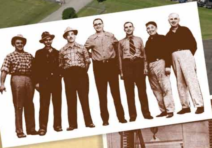
Behind the construction (L-R): W.I. Ritter, W.H. Wetzel, W.J. Sprau, P.J. Dumas, L.L. Hank, C.R. Cummings and L.E. Wilcox. The team was lead by S.D. Skinner from the "Home Office" of National Gypsum.
