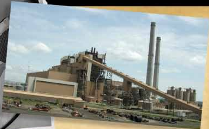
Another perspective on the GRDA Coal Fired Complex, which sits on a 1,245-acre site on the southern edge of MidAmerica. GRDA is a cost-of-service provider and public power utility.
