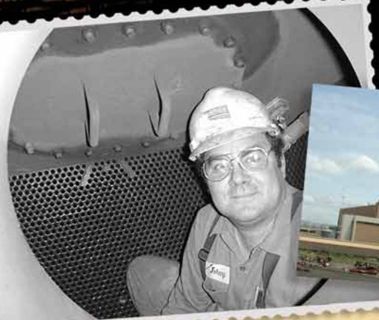
GRDA's Johnny Horn at work on the coal handling equipment at the Coal Fired Complex in the 1990's.
