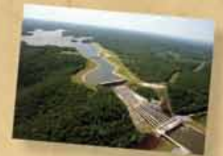
The GRDA Salina Pumped Storage Project, considered "experimental" during construction in the late 1960's, has a generation capability of 260 megawatts.
